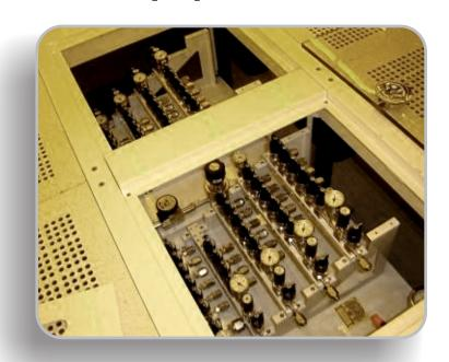
At NEHP, we are experts at all types of process tool & equipment installation. Shown here is an example of our patented (Patent # 7.039.999 B2), raised access floor (RAF), drop-in gas module for a semiconductor cleanroom. We can provide hookup needs or requirements for all utilities - electrical, mechanical, process gas, water, chemical, controls. etc.
