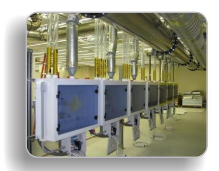
This turnkey piping system installation is a quality example of the onsite services performed by NEHP. We were contracted to design, install and commission the bulk chemical distribution system piping for a Solar Cell Manufacturing Facility. This system is all double-jacketed piping for Sulphuric Acid, Sodium Hypochlorite, Sodium Hydroxide, Sodium Sulphite & Sodium Chloride.
